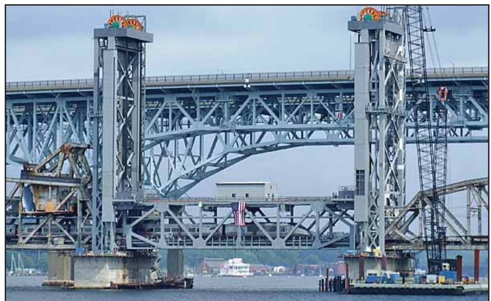
An Acela Express train crosses the new Thames River Bridge after completion.
